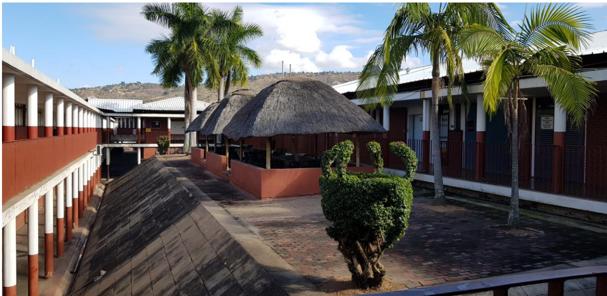
Foto 5: Themba Hospital – vnitroblok nemocnice
